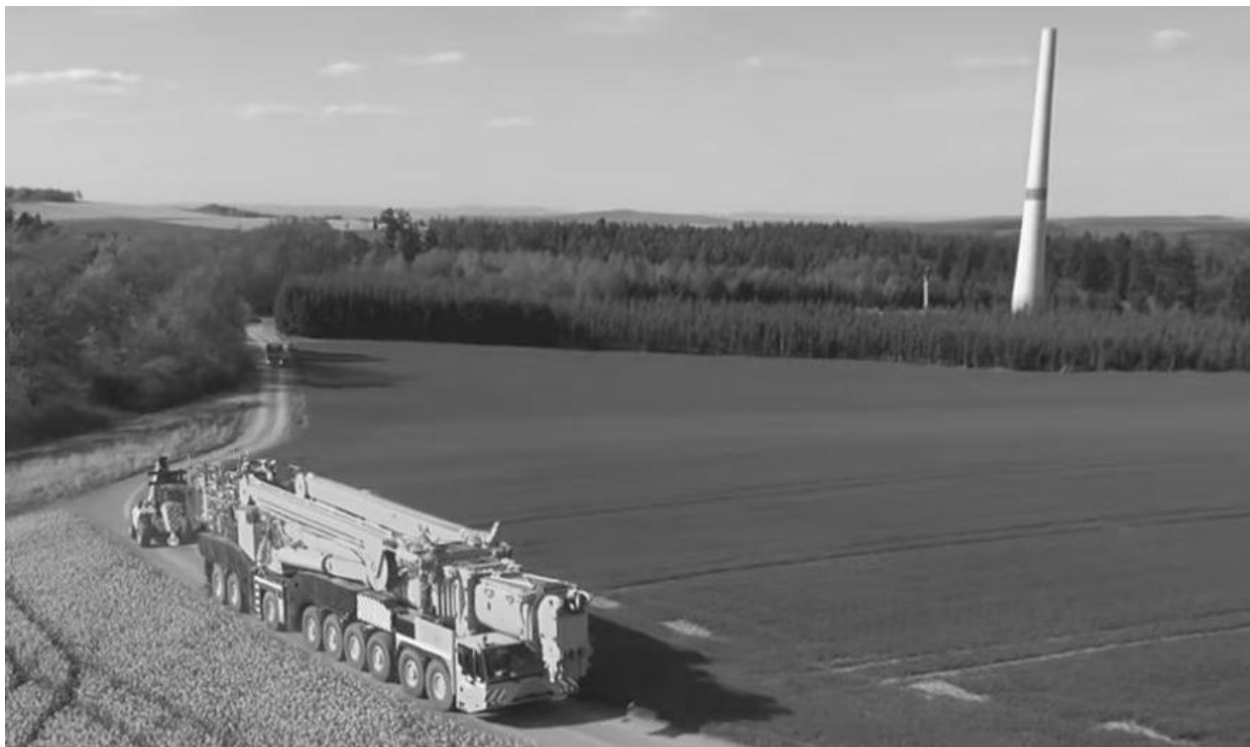
Example 3 – Nine-axle rubber-tired crane with partial counterweight and boom system installed
